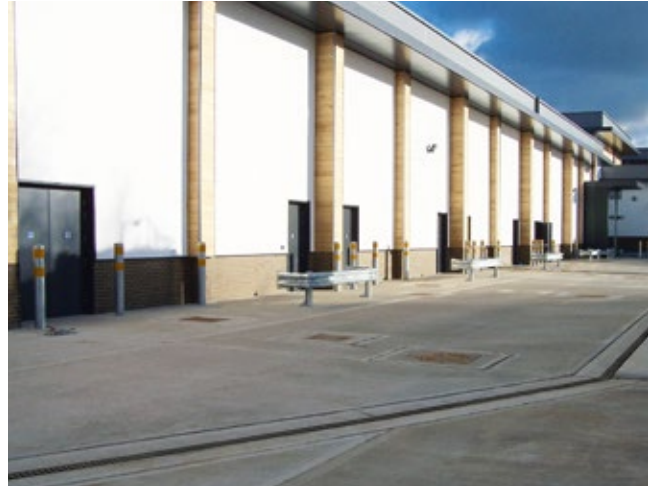
Installation in concrete surface
