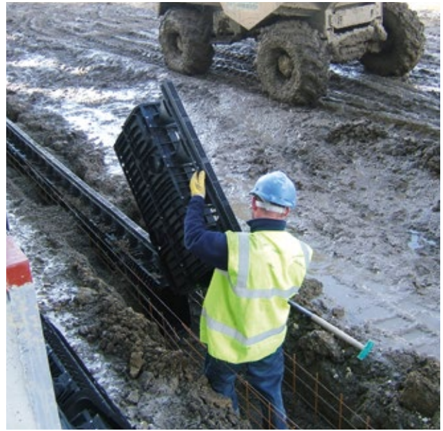
Lightweight elements, installed by one single worker.
