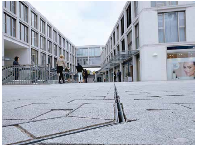
One of 50 tailor-made drainage channels.
