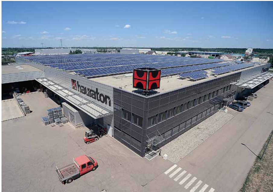
The major investment in a new plant at our headquarters is clear commitment to the Rastatt / Ötigheim location.
