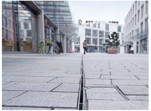
Surface drainage with tailor-made slotted channels.
